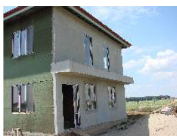
Figure 4 - External thermo insulation
