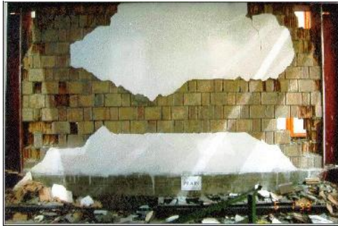
Figure 12 - Damage patterns for ordinary masonry
