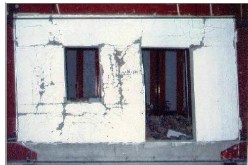
Figure 15 - Damage patterns for confined masonry
