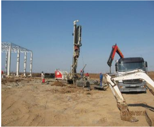
Fig. 2. The drilling process for the vertical earth loops.
