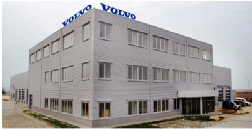
Fig. 1. Image of the studied building
