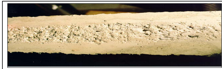
Fig.5 –Concrete surface after cleaning.
