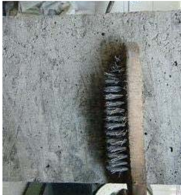
Fig.7 –Concrete surface after brush cleaning.
