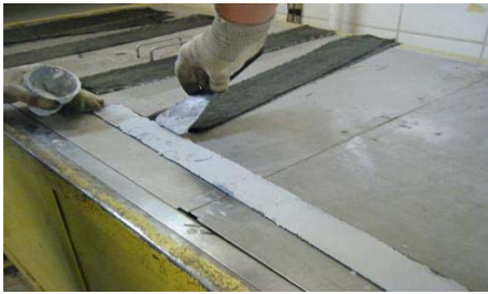
Fig.11 –Applying the adhesive.
