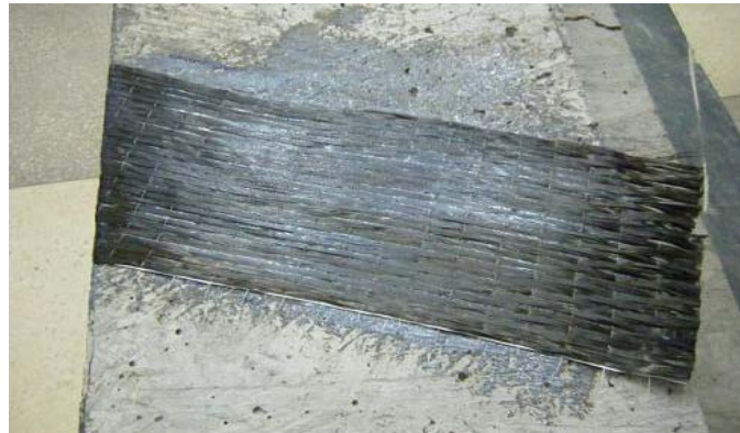
Fig.9 –The final aspect of CFRP sheets.
