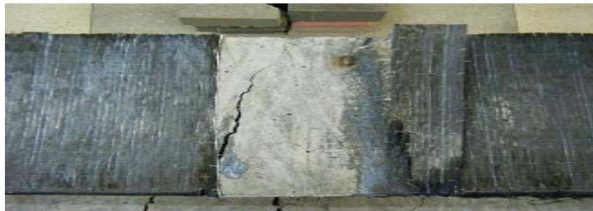
Fig.6. Position of crack for beam G3.
