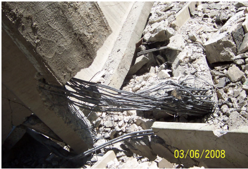
Fig. 3. Reinforcement of prestressed beams
