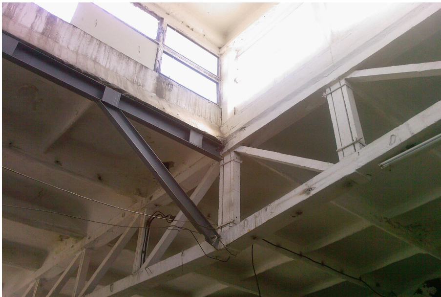
Fig. 2. Image before demolishing from the reinforcement workshop
