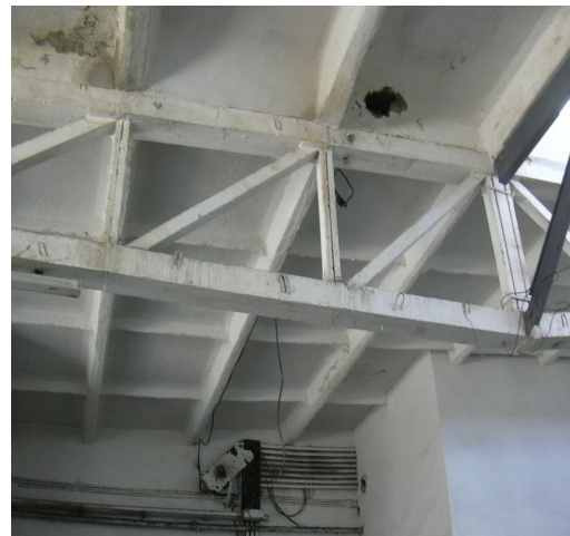
Fig. 6. The roof of workshop of reinforcement
