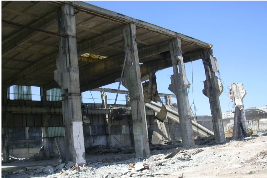
Fig. 1. Image of time shots demolishing from the prefabricated workshop.
