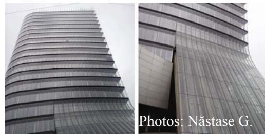
Fig. 12. UNIQA tower's double skin façade, Vienna, Austria
