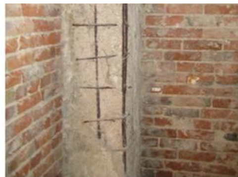
Fig.3. An existing pillar , at the basement of the building.
