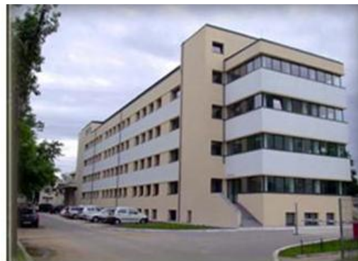
Fig.2. The building after rehabilitation
