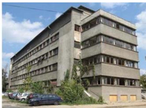
Fig.1. The building before rehabilitation
