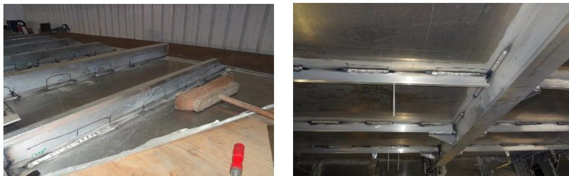
Figure 2: Welding of a luminium profiles
