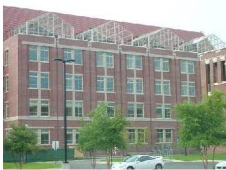
Figure 9. Greenhouses located on the roof of Florida State University [9]
