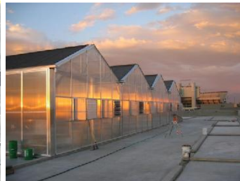
Figure 12. Greenhouse in Tucson, Arizona [12]
