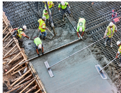
Fig. 3. Workers on pouring concrete
