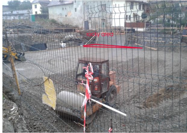
Fig 8. Image of the general excavation
