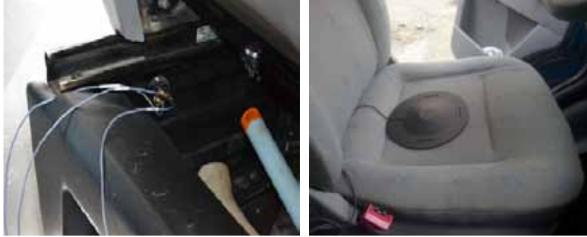
Fig. 6. Installation of vibration sensors type 4504 and 4447
