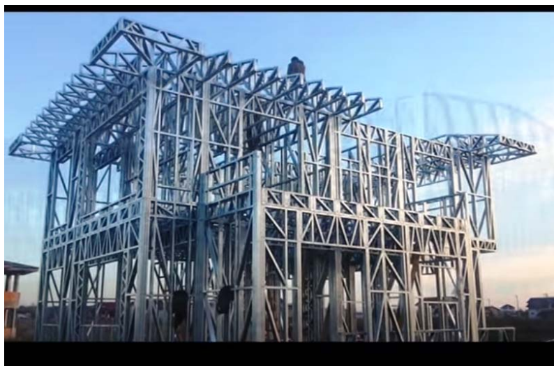
Figure 1: Lightweight metallic structure of building [2]
