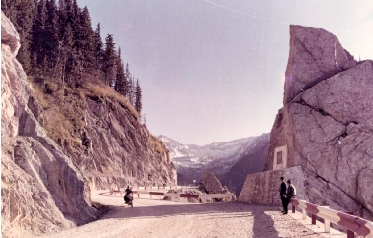
Fig. 2 Military Engineering Gate, km 25+320, Bălea Cascadă – Cascada Bălea road sector
