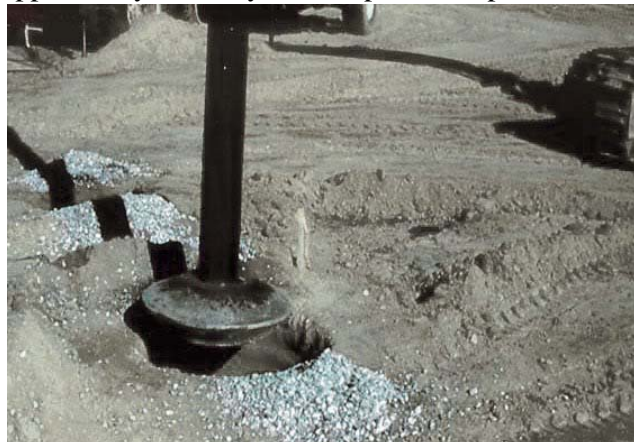
Fig. 1 Patented bevelled Geopier® tamper
