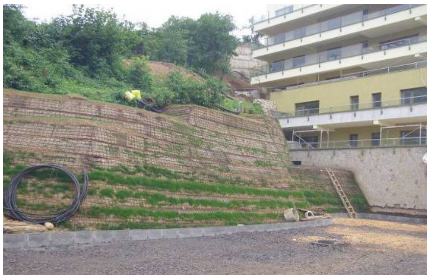
Fig. 24 – Soil structure ( H_e=7,00m )
