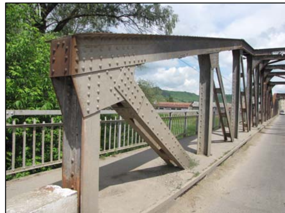
Fig. 7 Main truss girder
