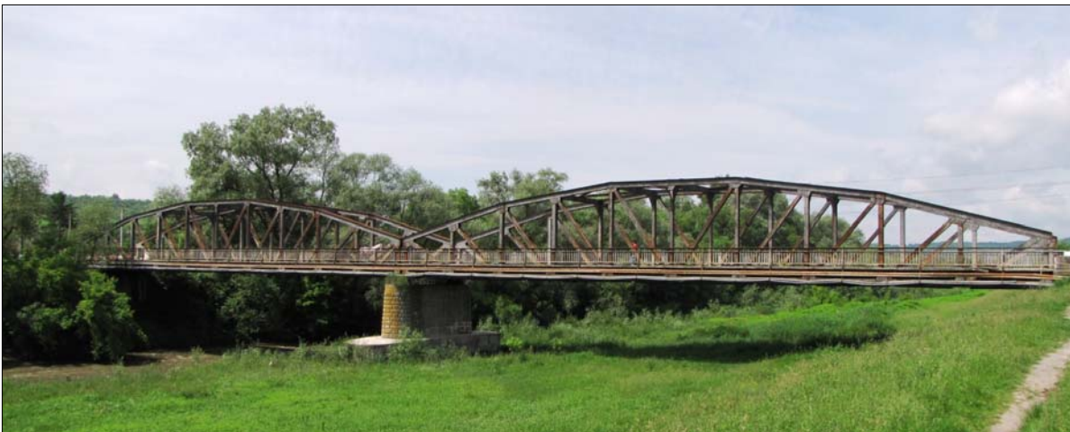
Fig. 4 General view of the bridge in Dumbrăveni
