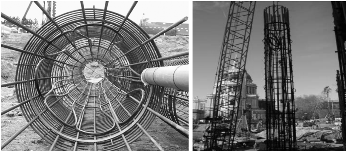
Fig. 4 Installation of geothermal tubes inside pile foundations [38]
