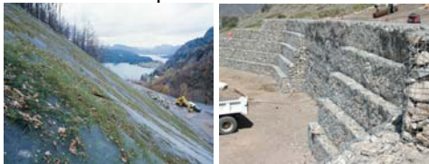
Fig. 3. Prevention of soil erosion and landslides
