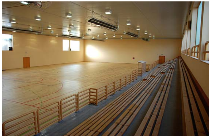
Fig. 6. Tested sports hall after completion
