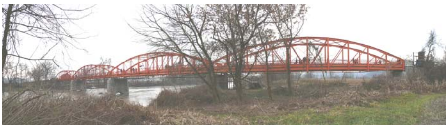
Fig. 6 Highway bridge in Săvârșin erected in 1897 and rehabilitated after 110 years in 2007
