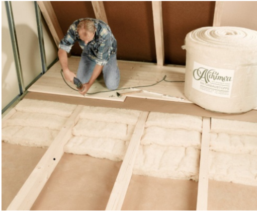
Fig. 11. Method to mount the cellulose fibers insulation
