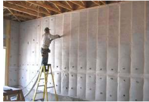
Fig. 11. Method to mount the cellulose fibers insulation
