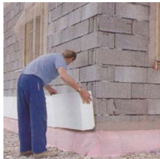
Fig. 9. The manner to put in place the expanded polystyrene
