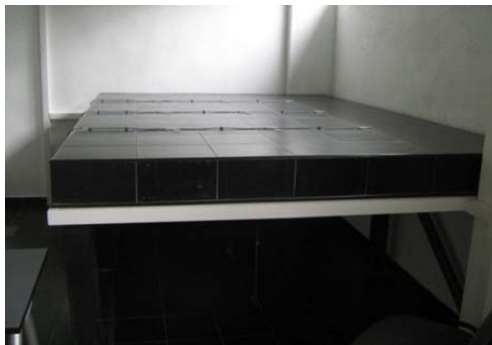
Fig. 1. TABS radiant surface in the faculty laboratory
