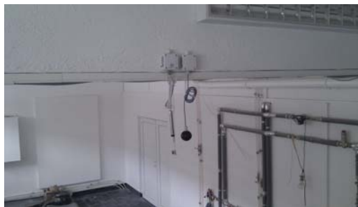
Fig.3 Sensors for measuring the relative humidity and radiant mean temperature.
