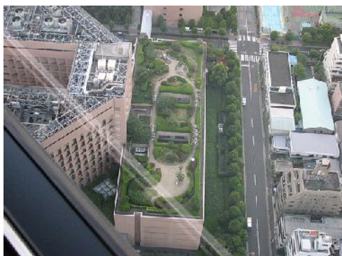
Figure 1: The roof of a hospital from Tokyo [1]
