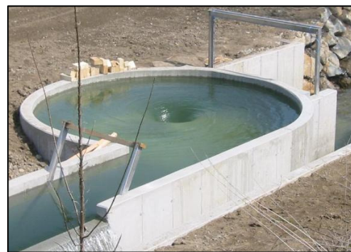
Fig. 3. Franz Zotlöterer's model of micro hydro facilities
