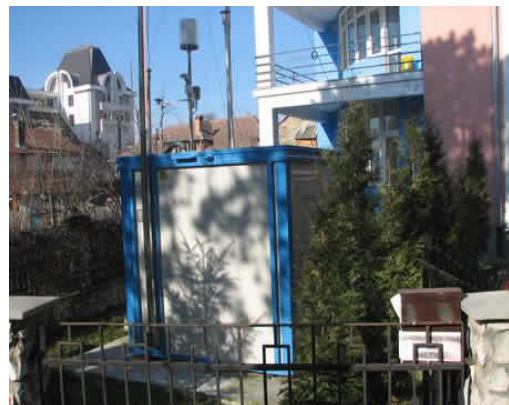
Fig. 3. Urban type monitoring station
