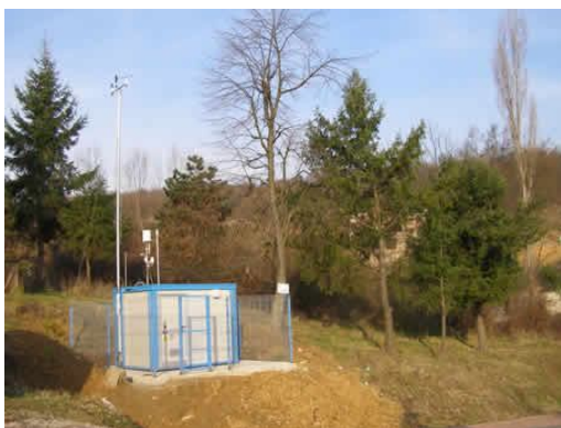
Fig. 6. EMEP type monitoring station
