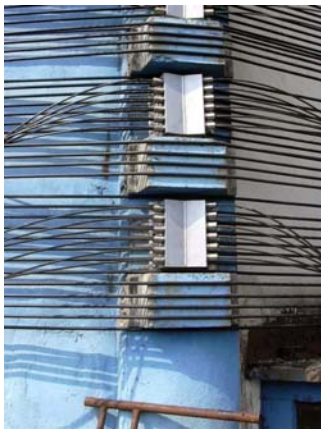
Fig. 9 Additional bearing steel blocs
