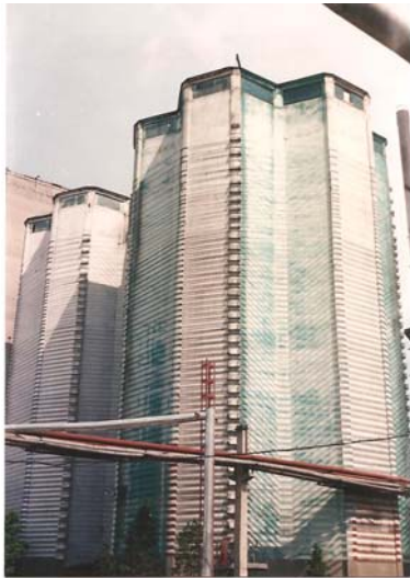
Fig.1 View of coupled silos
