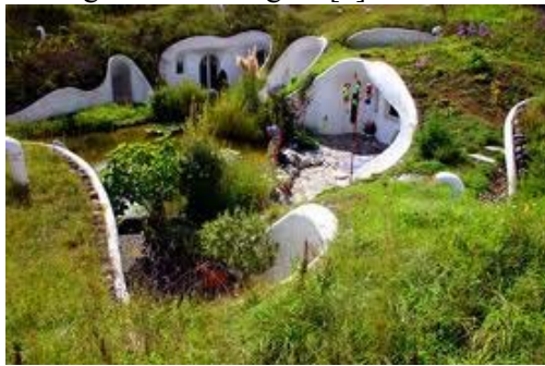
Fig. 3. Earth house - ecovillage
