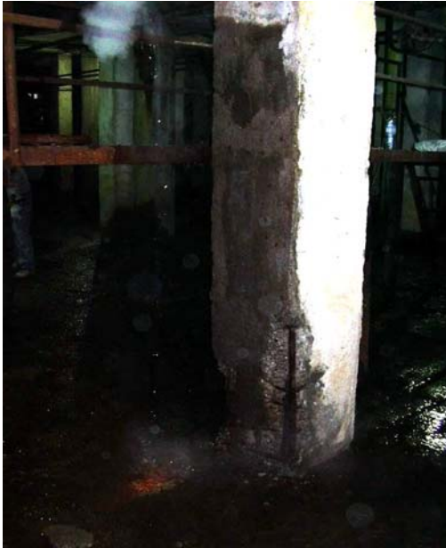
Fig. 4. Water pooling in the basement
