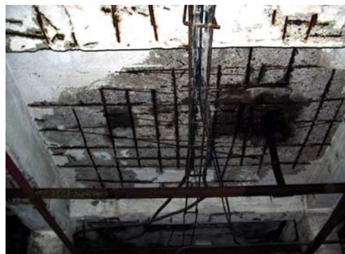
Fig. 3. Heavily corroded plate
