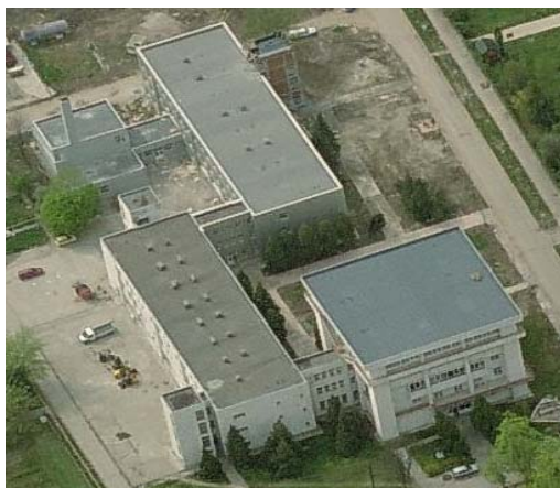
Fig. 4. The Faculty of Land Reclamation and Environmental Engineering in Bucharest
