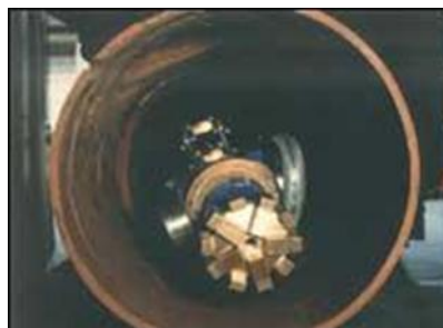
Figure 5: Pipe cleaning with the help of robots
