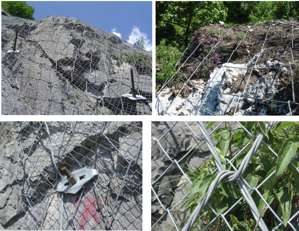
Fig. 2 Rock protection with high-tensile spiral rope nets combined with rock bolting
