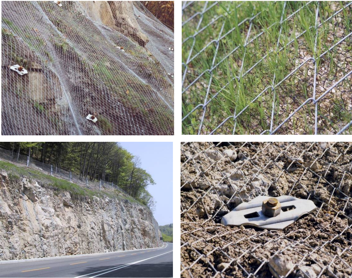
Fig. 1 Active stabilization of soil and rock slopes with high-tensile steel wire meshes in combination with soil nailing and rock bolting
