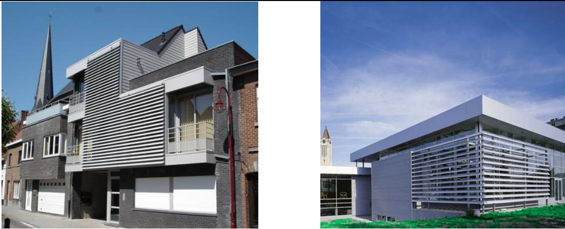
Fig. 5 Fixed oval section disks fitted.
