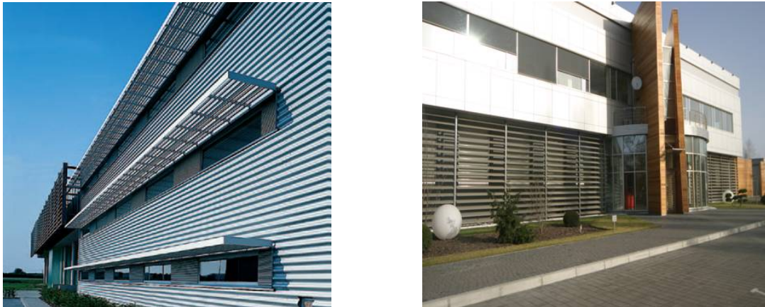
Fig. 2 Disks horizontally (left) and vertically (right) fitted.
