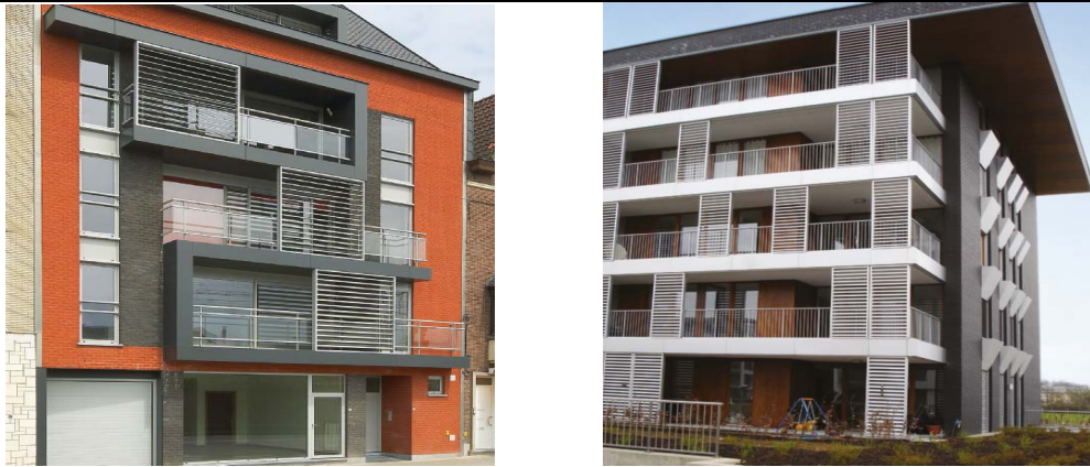
Fig. 8 External elements of solar protection made from mobile panels.
