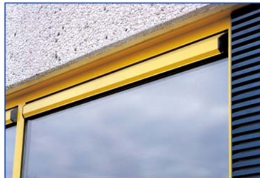
Fig. 3 Fan with air auto regulation flow according to the difference in pressure, indoor-outdoor.
