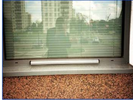
Fig. 8 Fan mounted into the window frame.
