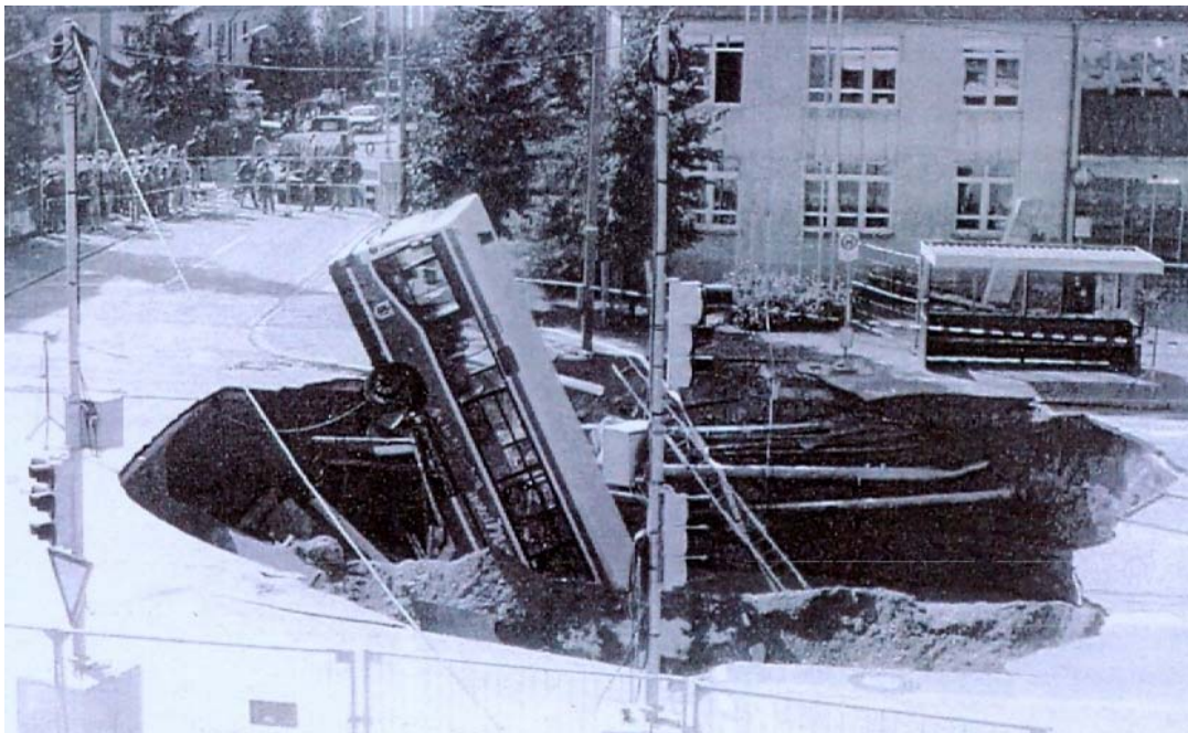
Fig. 3 Consequences of choosing the wrong technology or non-compliance. Tunnel in Munich-Germany 1994
