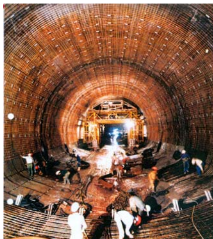
Fig. 2 Tunnel NATM method executed.
