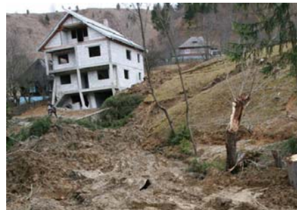
Fig.2 Landslide (Maramures, Romania)
