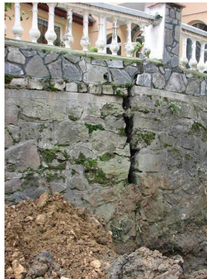
Fig. 3 The large opening of the compression joint
