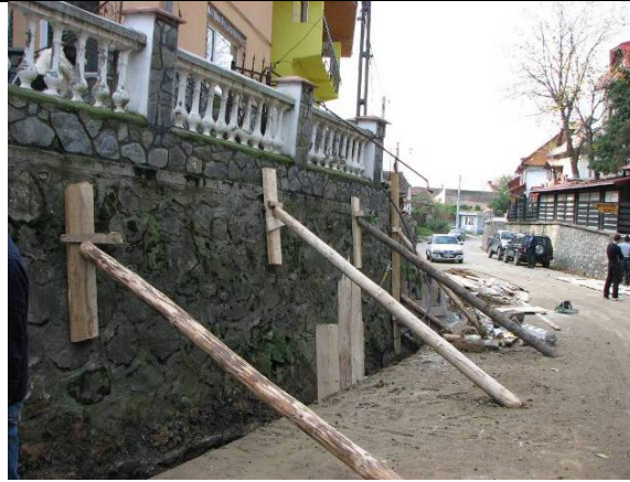
Fig. 2 The digging carried out on long sections near and under the foundation quota of the retaining wall
