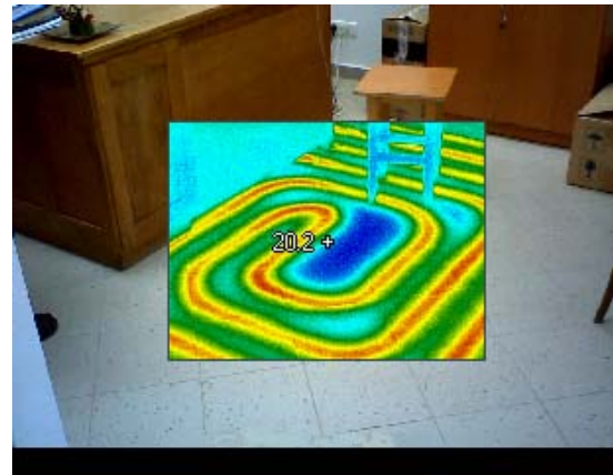
Fig. 3 Thermo vision of the hydronic circuit
