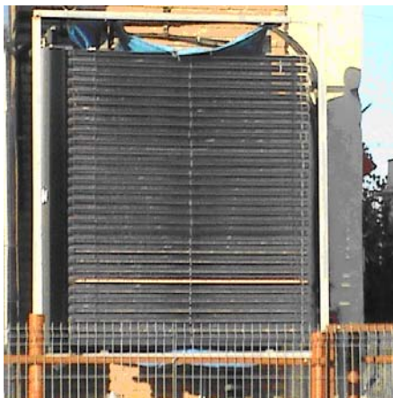
Fig. 5 The evacuated solar collector
