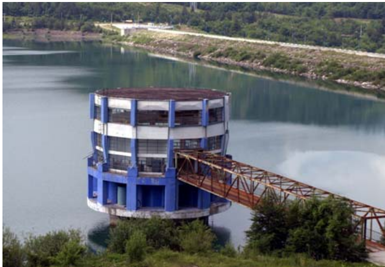
Fig.1. Water intake from the Sacele accumulation
