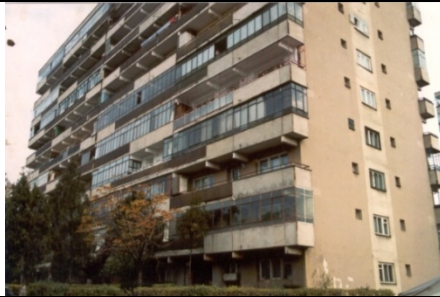
Fig. 2.3. PLOIEȘTI – WEST, 149 C Bldg., PLS
