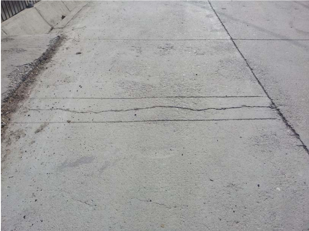
Fig. 4. Transverse cracks
