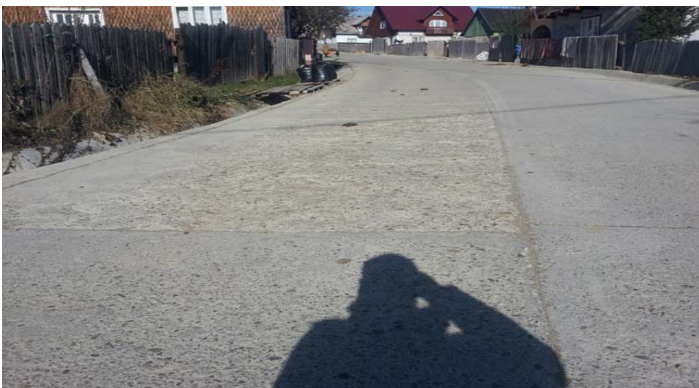
Fig. 3. Exfoliation of the surface
