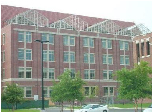
Figure 5: Greenhouses placed on the roof of the Florida State University [4]
